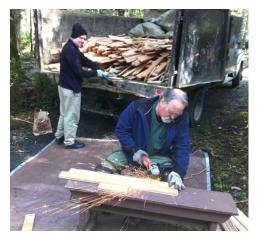
After a lot of research on what to put on the floor (over the plywood foundation) we decided to buy some oak hardwood flooring from craigslist that was being removed from a house slated for demolition. This was a huge undertaking, as the flooring had to be loaded onto a truck, transported to Kitsap, unloaded from the truck – and every piece had to have all of the nails grounded out.
