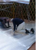
The second day was the fabric installation. Every seam (front and back) of all three layers of roof insulation had to be taped with a special silver tape – a 3 to 4 hour job.
