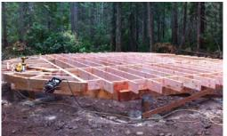
October 17<sup>th</sup> the concrete was delivered and poured into holes. Even this caused an emergency call to Mike Bonomo to cut down a small evergreen in the way of the cement truck.
