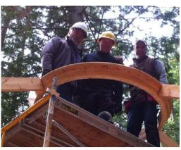
After all 44 rafters were installed, wood braces were installed between each rafter pair (half high and half low). This was probably the most tedious part of the job. The happy crew poses after day one of work.
