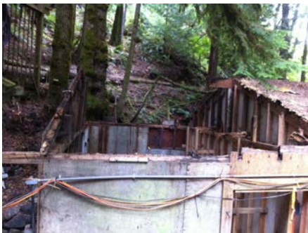
more rotten wood to be removed on wall
