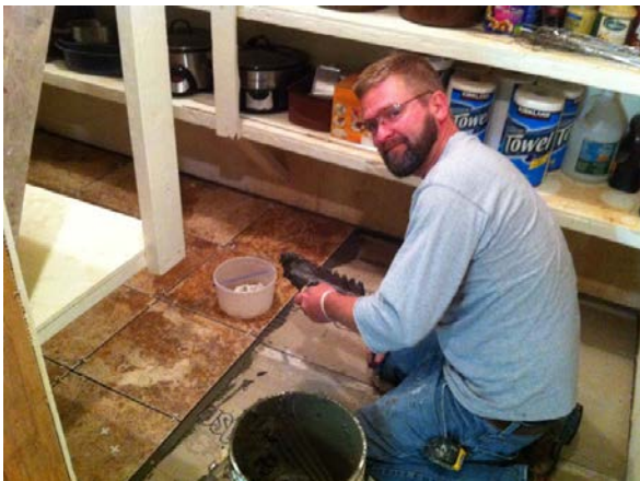
Mark McNeill tiling the pantry
