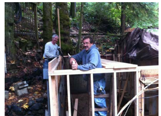
Steve and Vince working on the new roof joists
